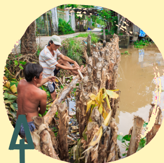
After receiving construction materials and technical training as part of the Foundation's ACCCRN work, local community members take flood prevention into their own hands, constructing several kilometers of erosion barriers along the riverside.
