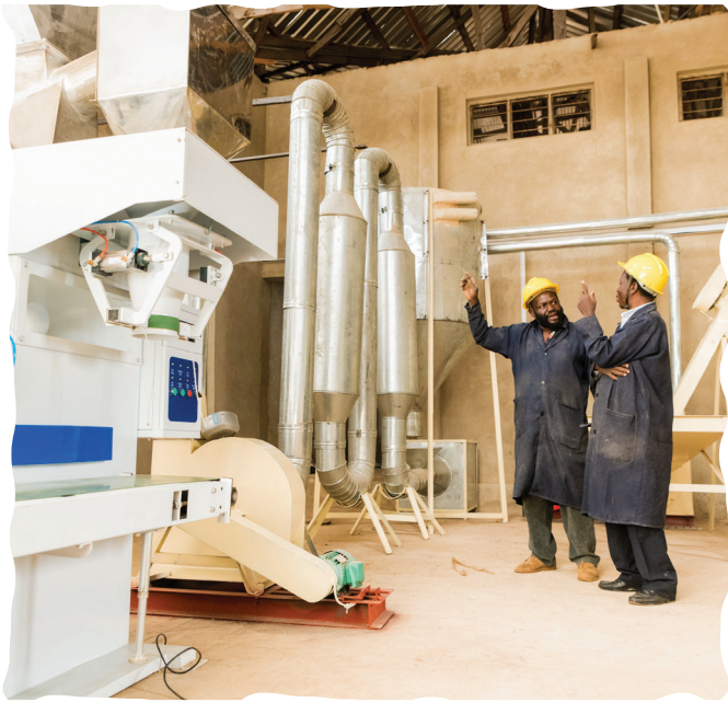
Installation of the new plant is almost complete.
