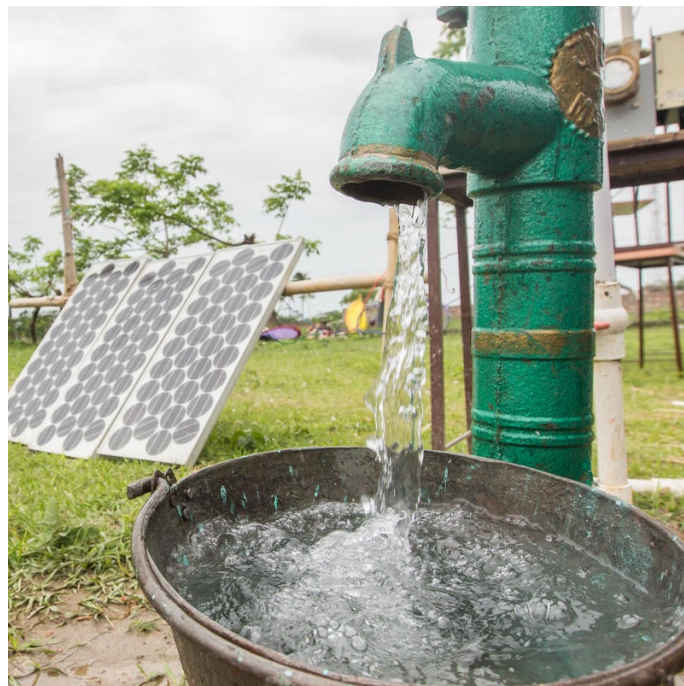
A SOLAR-POWERED PUMP ENABLES USERS TO DRAW WATER WITHOUT HAVING TO MANUALLY PUMP THE HANDLE IN GAYARI, ARARIA DISTRICT, BIHAR, INDIA. PHOTO COURTESY ROCKEFELLER FOUNDATION
