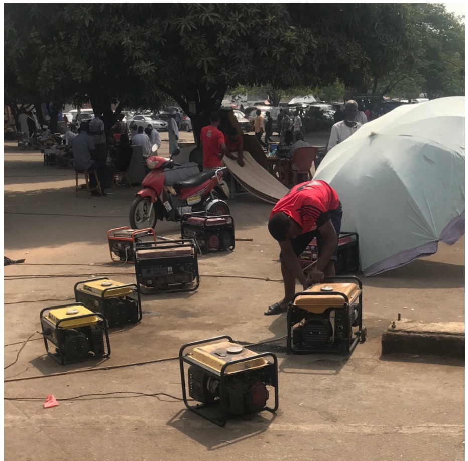
PORTABLE GENERATORS IN USE AT WUSE MARKET , PRIOR TO INSTALLATION OF THE MINIGRID SOLUTION
