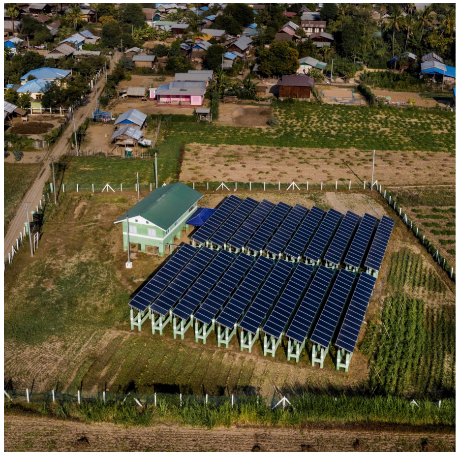
A SOLAR MINI-GRID IN SE PIN KYUN VILLAGE, SAGAING REGION, MYANMAR. PHOTO COURTESY SMART POWER MYANMAR
