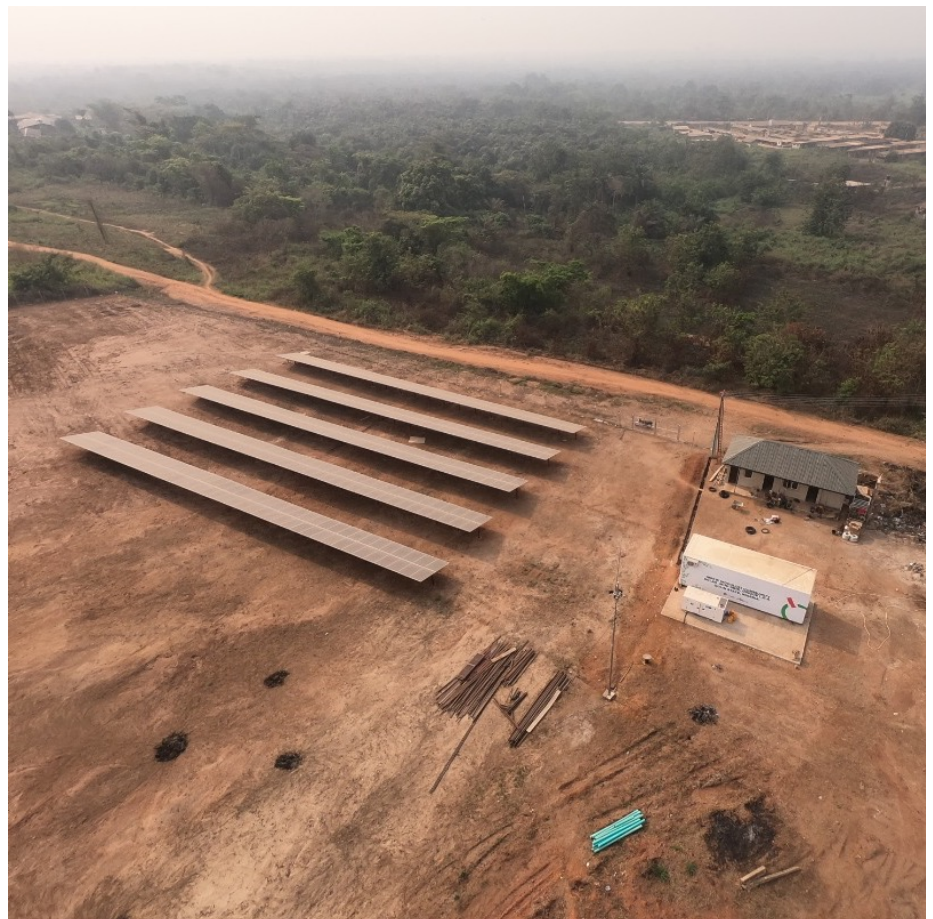
MOKOLOKI MINIGRID, OGUN STATE, NIGERIA (UNDER CONSTRUCTION)
