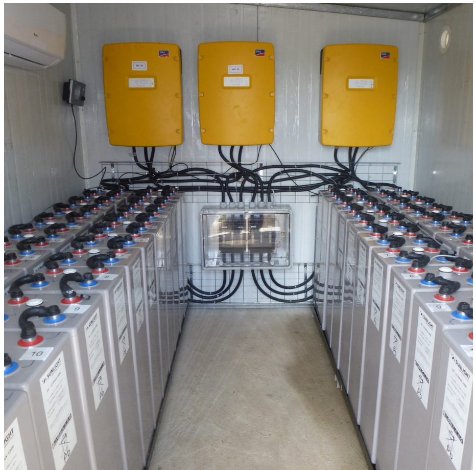
BATTERIES AND INVERTERS ON A MINIGRID IN SIERRA LEONE. PHOTO COURTESY INENSUS
